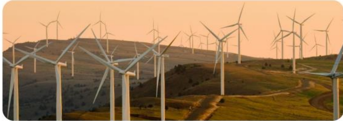
Twenty 5MW wind turbines
